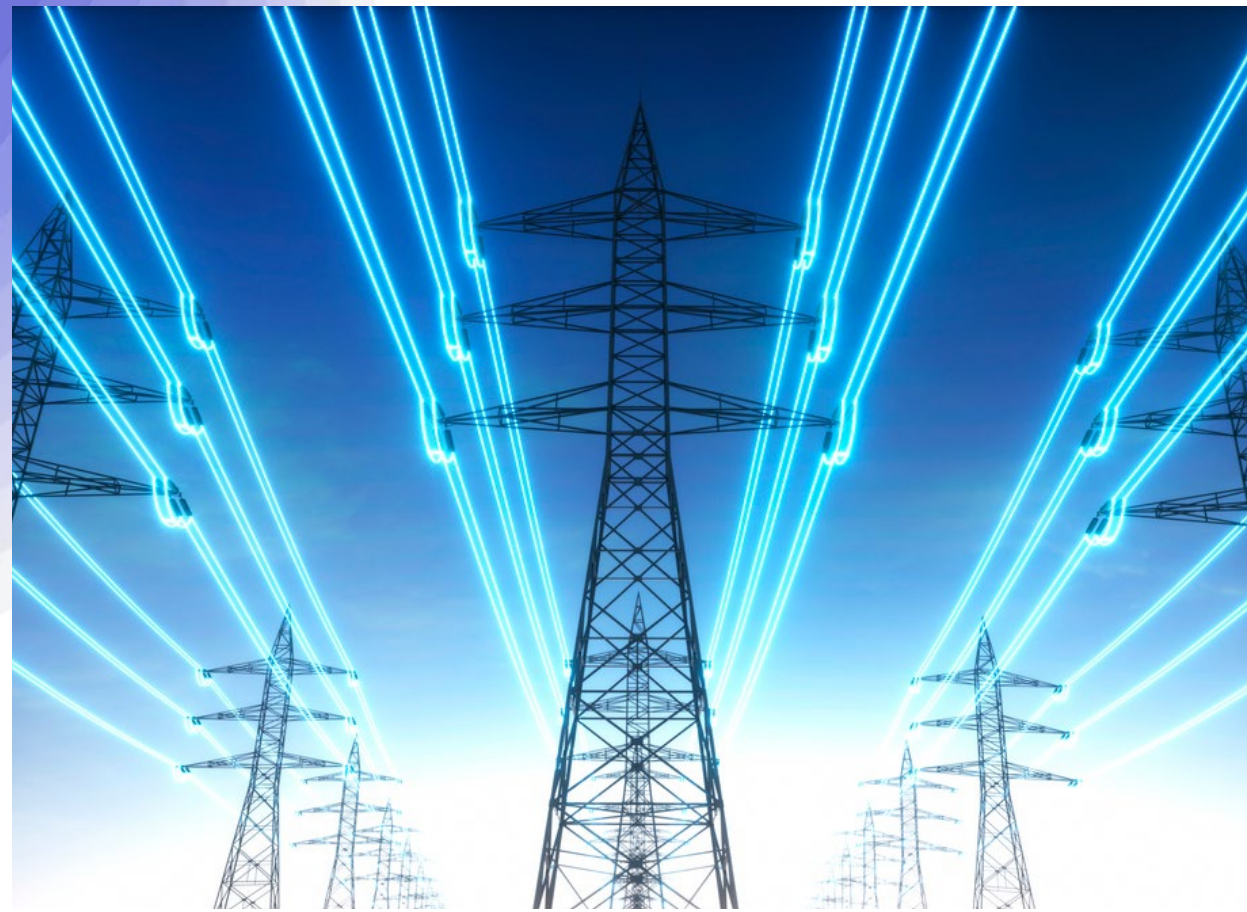
Ultra high voltage power lines are needed to effectively distribute energy from renewable resources.
