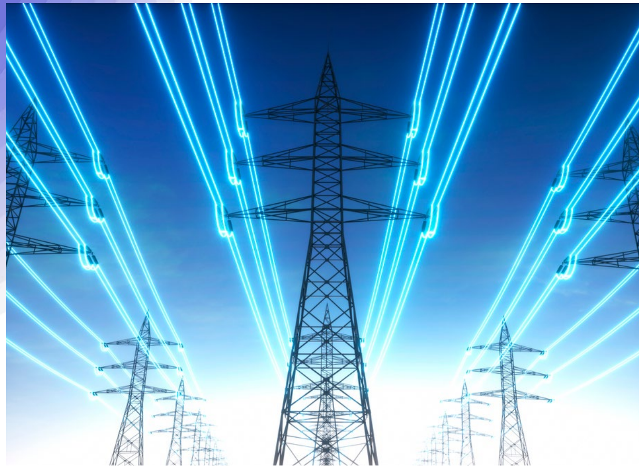
Ultra high voltage power lines are needed to effectively distribute energy from renewable resources.
